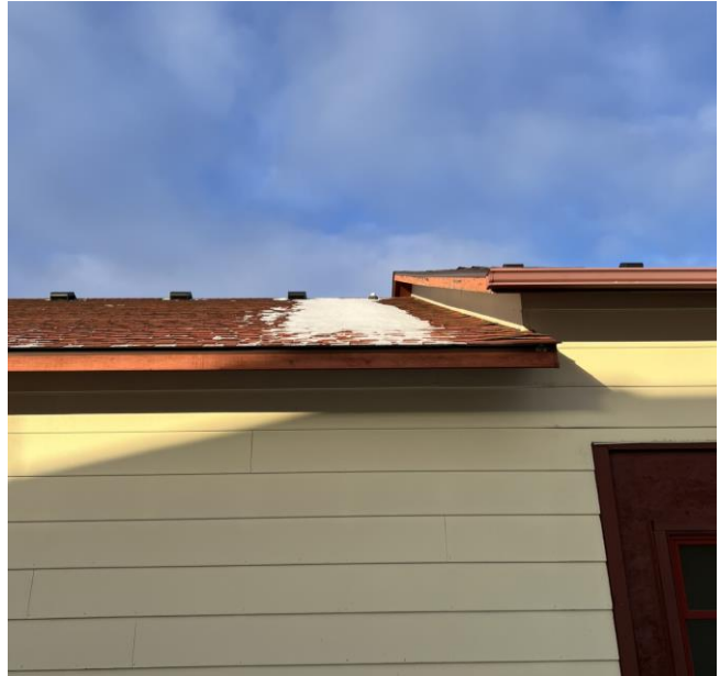
Asphalt Shingle Roof
