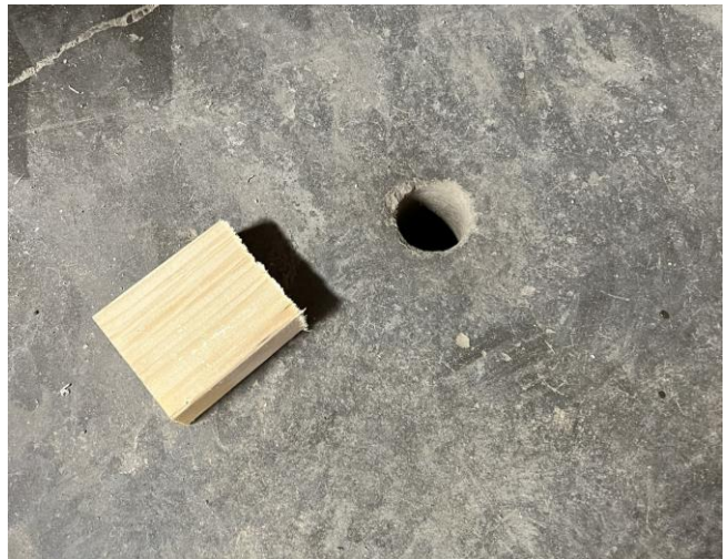
Hole in concrete slab for drainage
