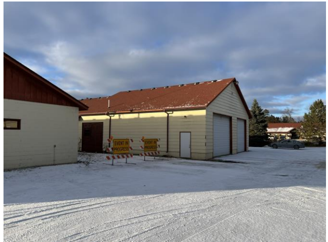
Asphalt Shingle Roof
