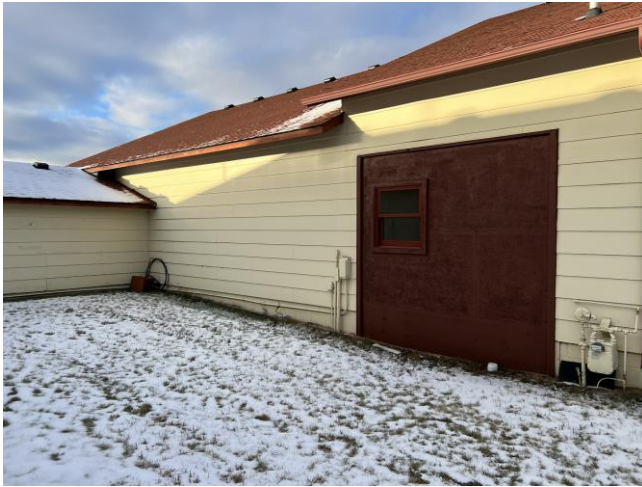
OSB Infilled opening
