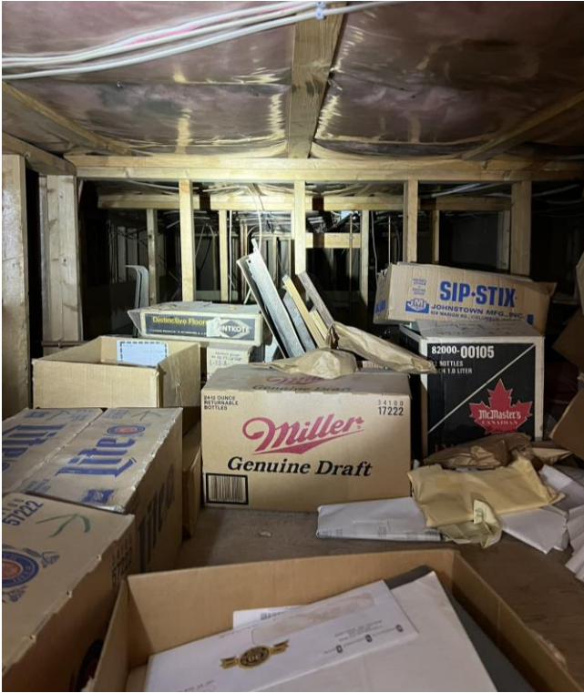
Cavity space currently being used for storage
